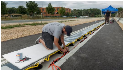
Figure 7. Setting the coil in the path [13]
