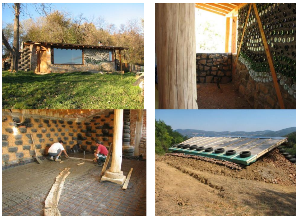
Figure 5. Car tyre house in the village of Brusnica near Gornji Milanovac
