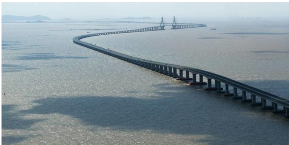
Figure 3. Dayang-Kunshan Grand Bridge
